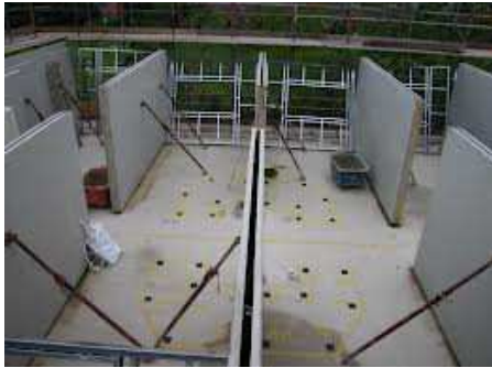
wallpanels with temporary supports
