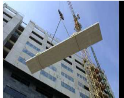
lifting slab panels
