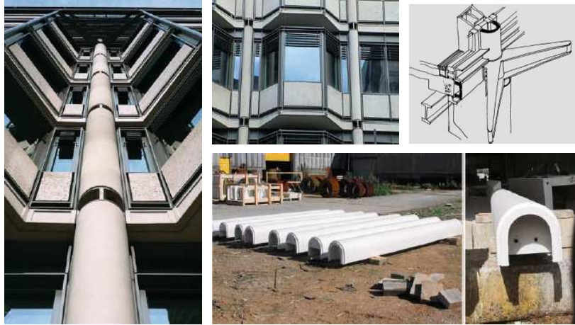
GRC facade wall elements, Office building, 25 – 35 Park Lane, London, United Kingdom
