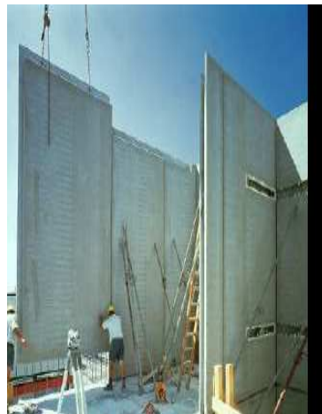
lifting wall elements
