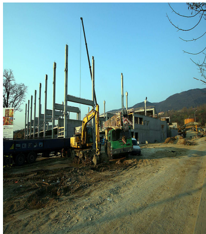
erecting multi-storey pillars
