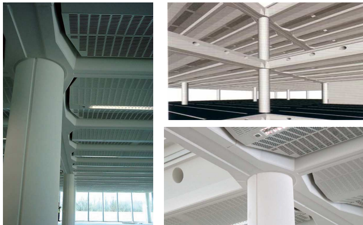
SCC construction elements, Office building, 35 Homer Road, Solihull, United Kingdom
